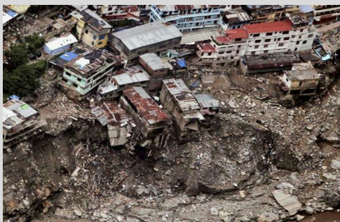
Figure 2: Consequences of the landslide in northern India.
